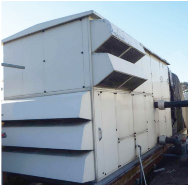
Unit condition before
