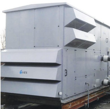
Completed refurbished unit
