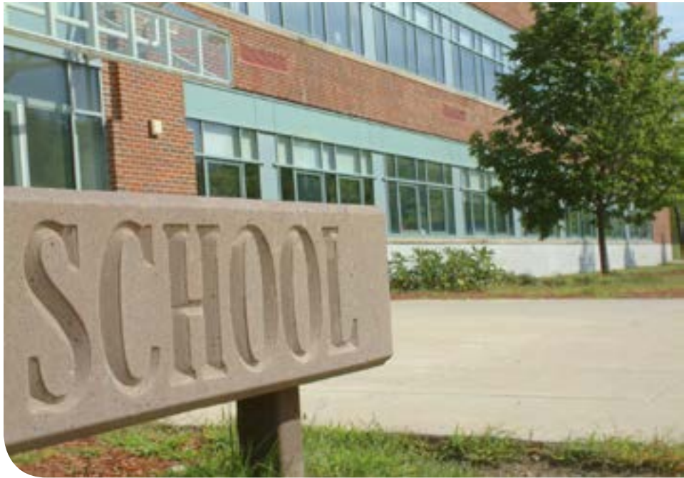
Changes for ventilation in schools
