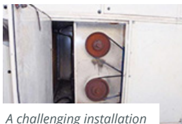
A challenging installation
