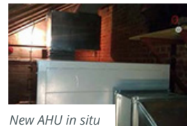
New AHU in situ
