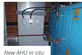
New AHU in situ
