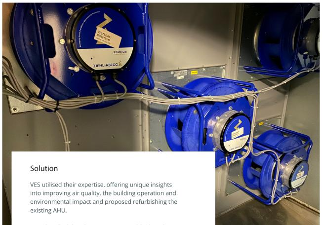
VES identified that the maximum possible duty the existing unit was capable of achieving was 10.7 m³/s due to maximum velocity limitations over the existing components. VES proposed 5no EC plug fans to work simultaneously in a fan wall to achieve the new increased design duty.
