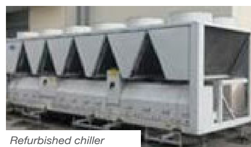
Chiller re-installation
